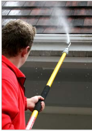
We'll leave your fascias, soffits, gutters, downpipes and drains spotlessly clean.
